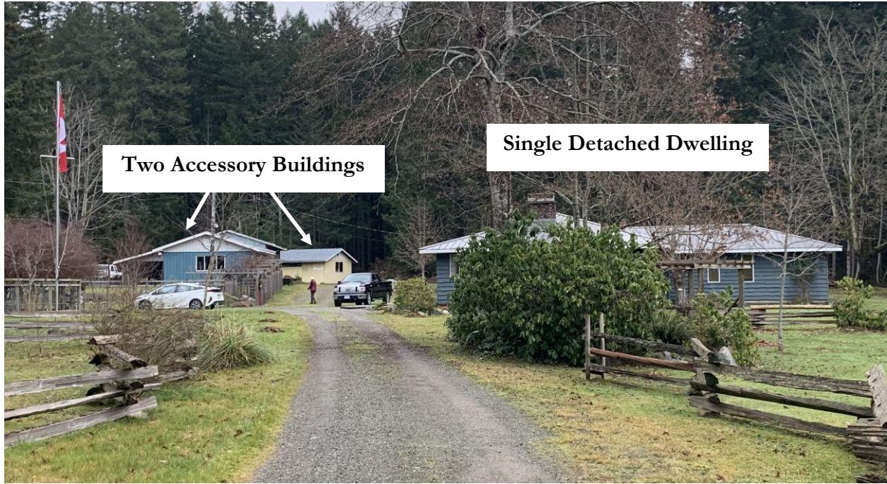
Figure 4: View of the Buildings from the Driveway
